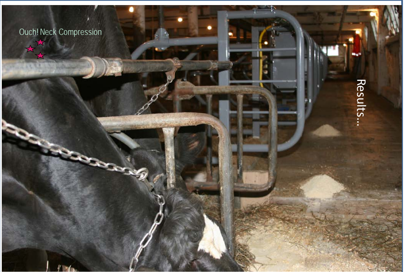
Junction of old and new – front view. Note height and forward position of neck rail
