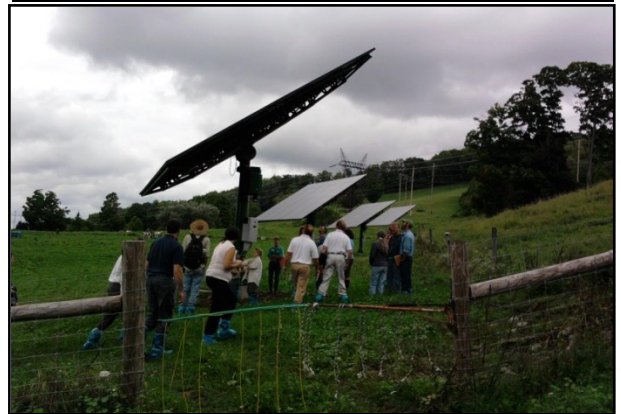
Participants at the Farm Renewable Energy Field Day at Twin Oaks Dairy LLC in Truxton, NY look at the 4 "trackers" that supply electricity to the farm and its 2 households.
