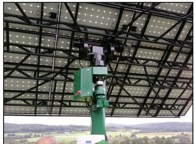
The underside of one 30-panel "tracker." This shot shows the 2 axis system – one rotates around the black axle daily, while the other swivels from left to right (or right to left) as seasons change.
